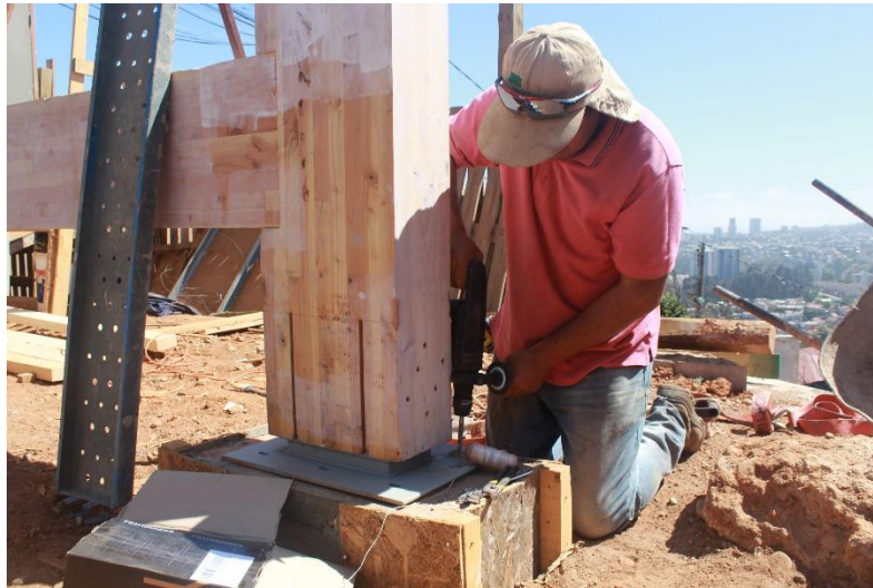
Figure 6: Frame instalation, column metal connectors with concrete foundation.
