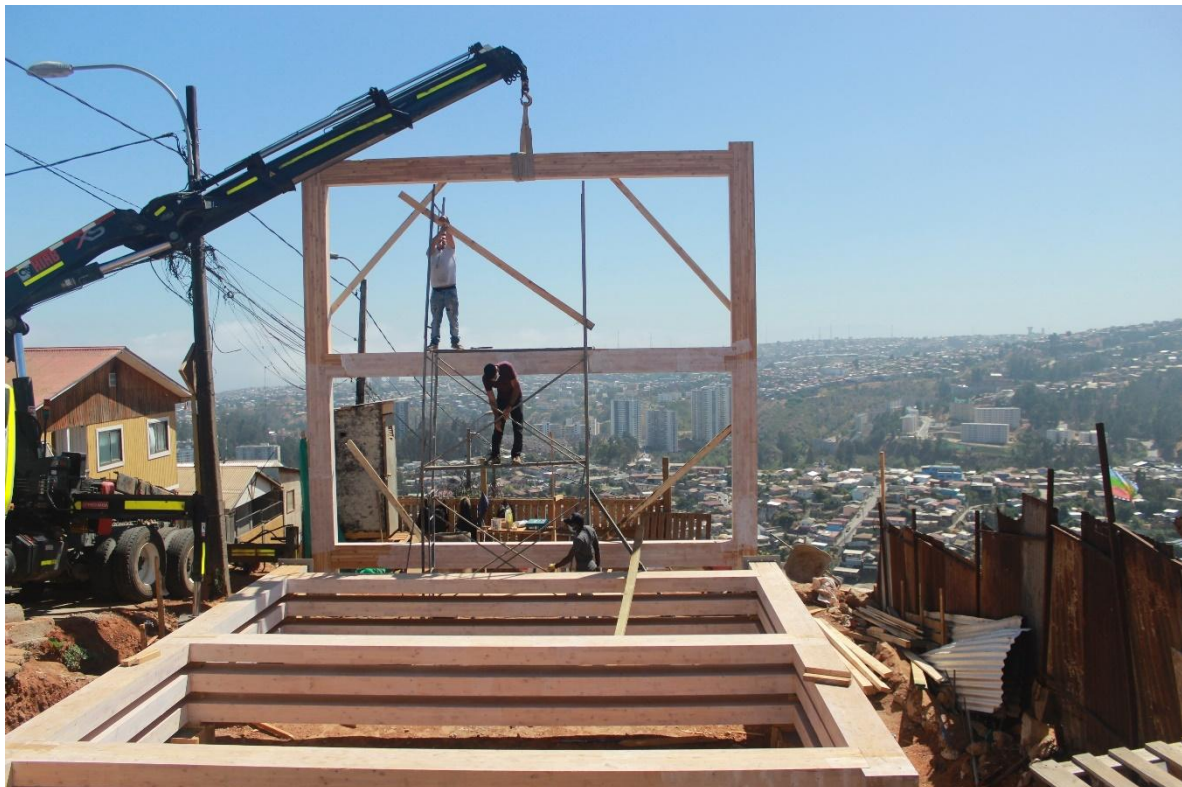
Figure 5: Lifting of the first structural frame.
