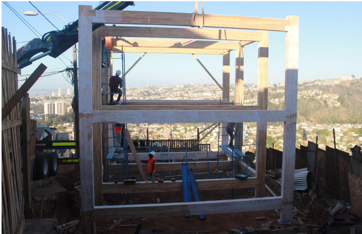
Figure 7: Complete lifting of the four frames of the main structure.
